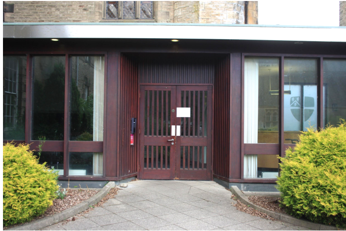
The East Wing Entrance - Fully Accessible/ Level Access
